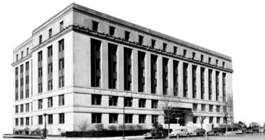
Figure 2. Envelope condition prior to retrofitting
